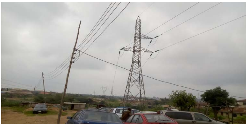
Figure 1. Automobile mechanical workshop under 330/220 kV power transmission line in Osogbo.
